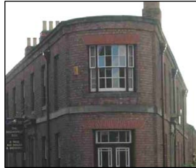
Examples of Tripartite vertical sliding sash windows
