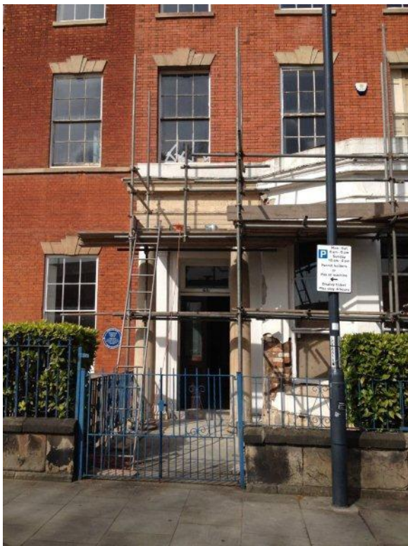
Top left Cleaned columns and portico exposing high quality stonework Top right exposed stone column behind bay Below exposed bricks not attached to original Georgian Stonework to rear
