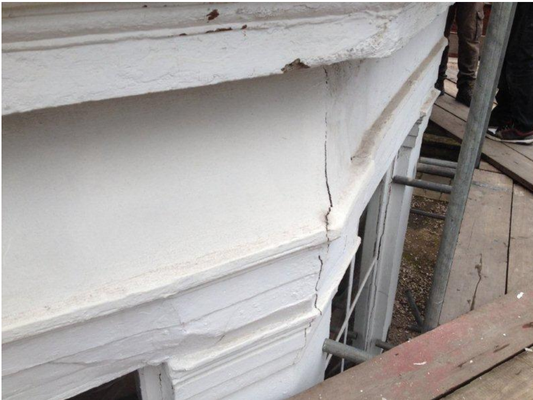
Modern Repair to clay element above at junction with stone of original portico and failing below
