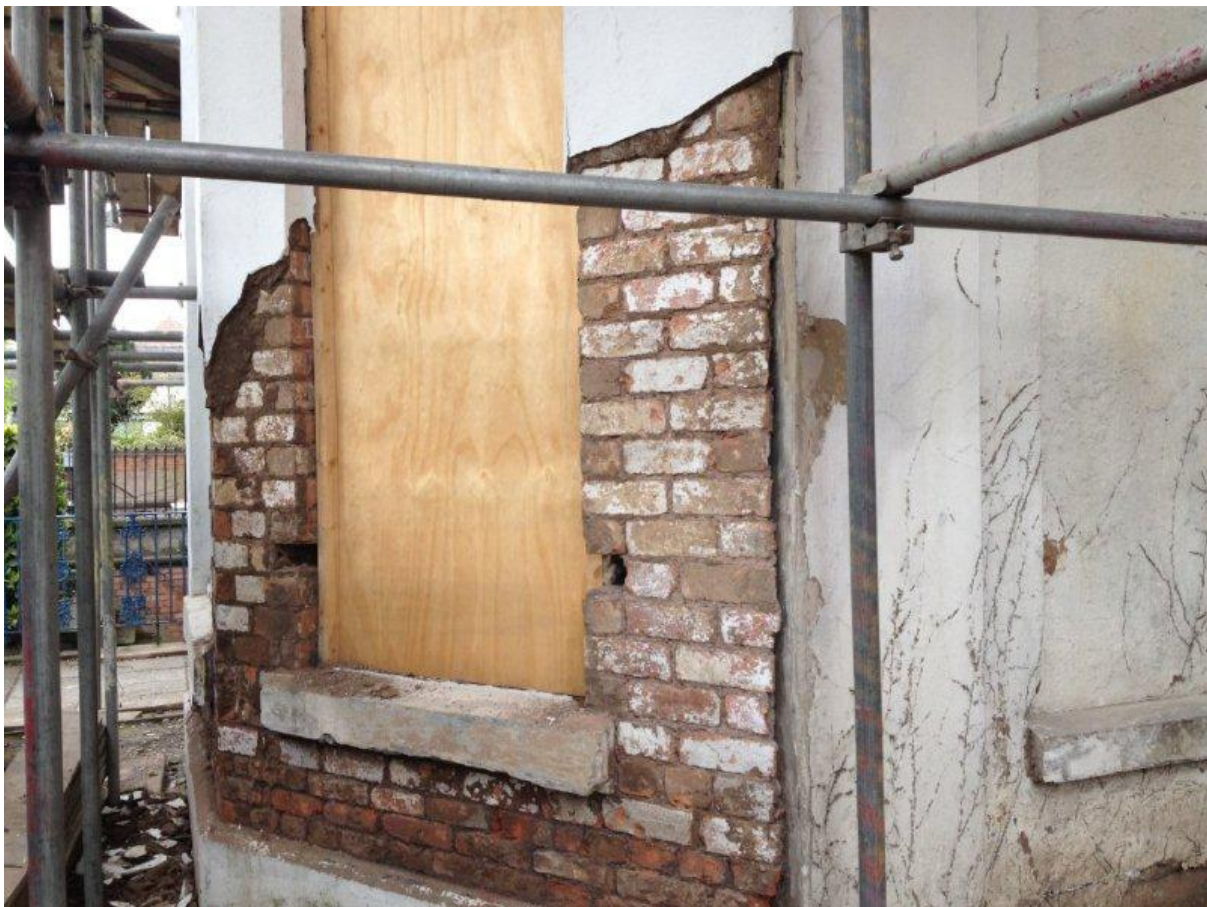
Top left Cleaned columns and portico exposing high quality stonework Top right exposed stone column behind bay Below exposed bricks not attached to original Georgian Stonework to rear
