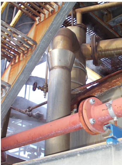
Photograph 2 Benzene Storage Tanks C17 - Vent for Down Pipe
