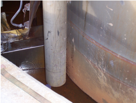
Photograph 1 Benzene Storage Tanks C17 and C17B - Venting Into Bunds
