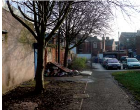
Unsecured rears to properties and dumping of rubbish
